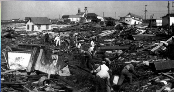
Significant damage caused by surge in Holgate, NJ during the Hurricane of 1944.
