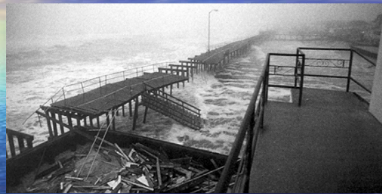
December 1992 Nor'easter destroys a section of boardwalk in Ocean City, NJ.
